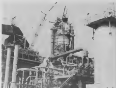
Two refinery units are undergoing major turnarounds. Above: the vacuum tower during the V3AR turnaround activities. Below: employees are inspecting the new pigtaills at the H3AR unit.
